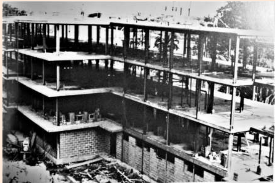
1New dorm under construction
